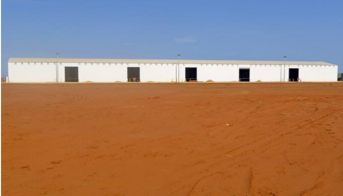
Figure 12. Ammonium nitrate storage shed
