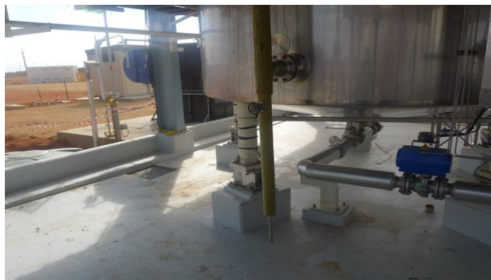
Figure 17. Concrete bunding and sump
