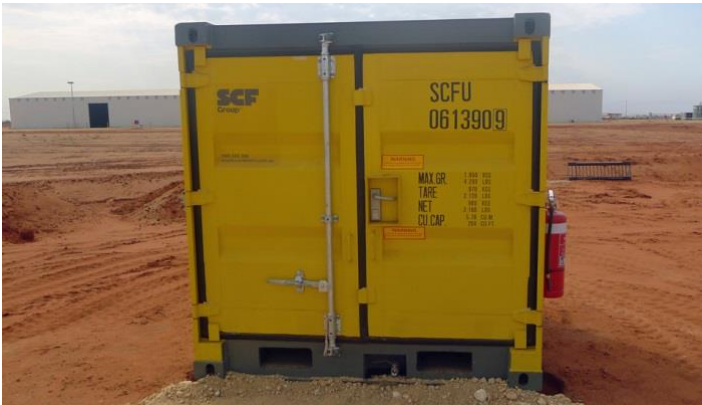
Figure 14. Flammable goods cabinet
