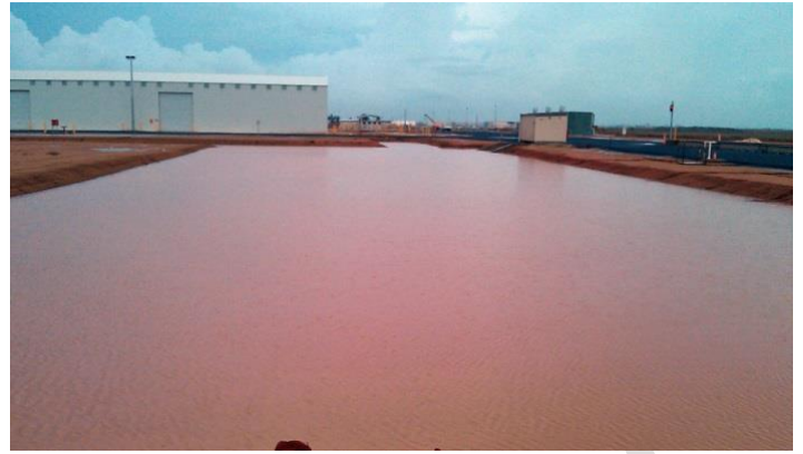
Figure 21. Stormwater retention pond
